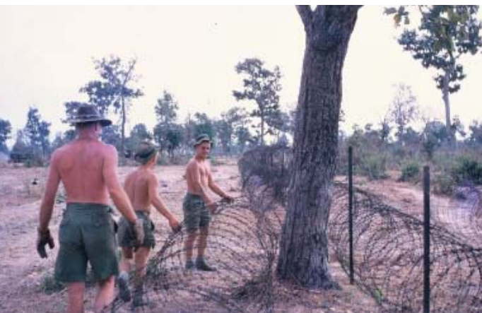
Sgt Jack Brown and Spr s Humphrey Dodd and Darryl Hess erecting the perimeter fence at the main camp site.
