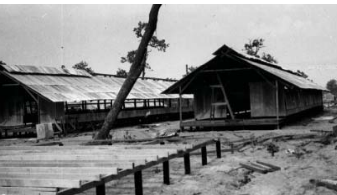
Barrack hut based on a design by WW2 Australian Army Engineer in Chief, Major General Sir Clive Steele. It is doubtful that Sir Clive would have been impressed with the finished product.
